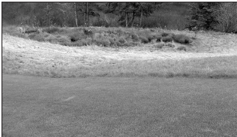
Grass buffer and artificial wetland designed to filter contaminants from water before flowing into natural wetland and lake.
